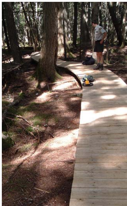
Assessing ground cover regeneration following boardwalk installation (photo by D.Ure, Parks Canada).
