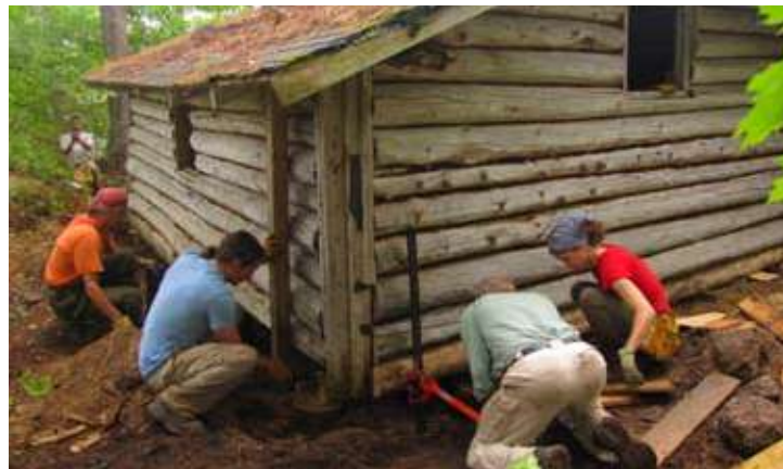
Log builder and volunteers jacking the cabin up out of the ground
