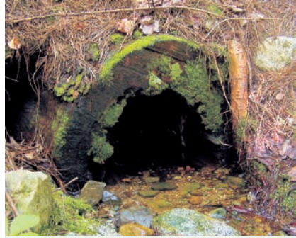
Hemlock culvert, Lake Rossignol
