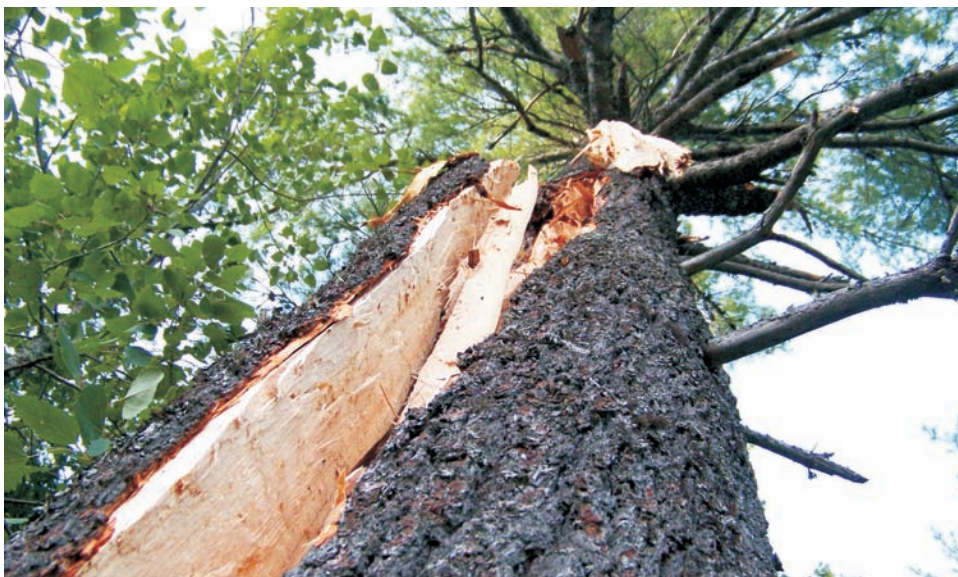
Lightning damage, Maitland Bridge
